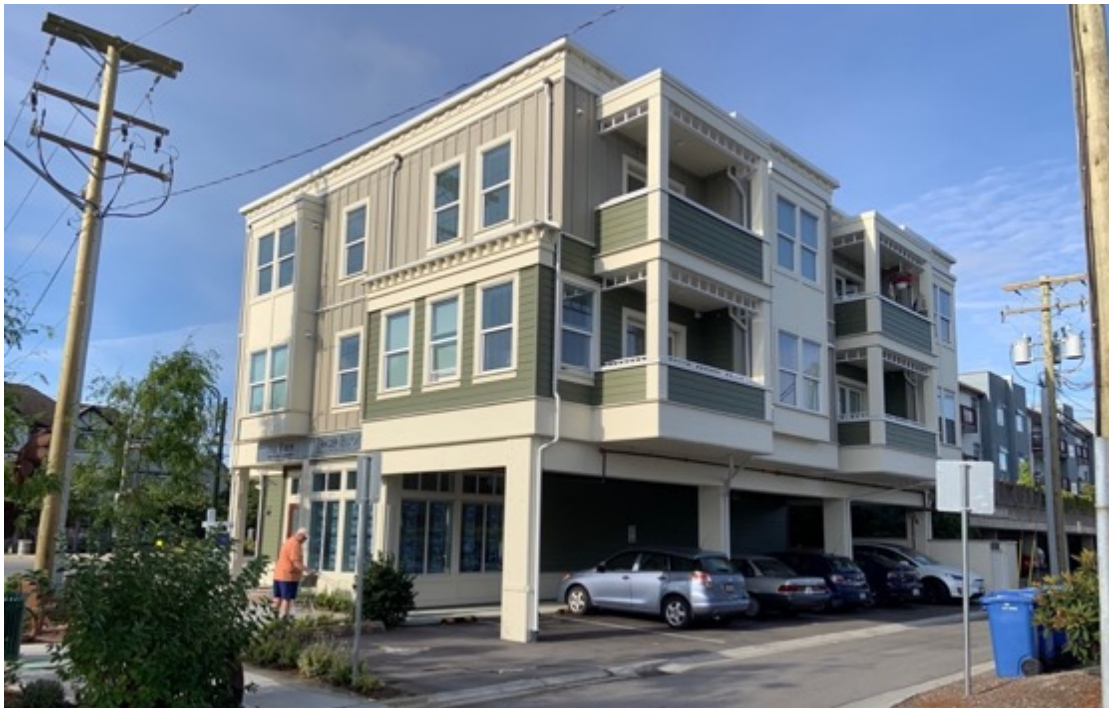
New three-storey mixed-use building with retail on first floor and residences above in Ladner, BC.
