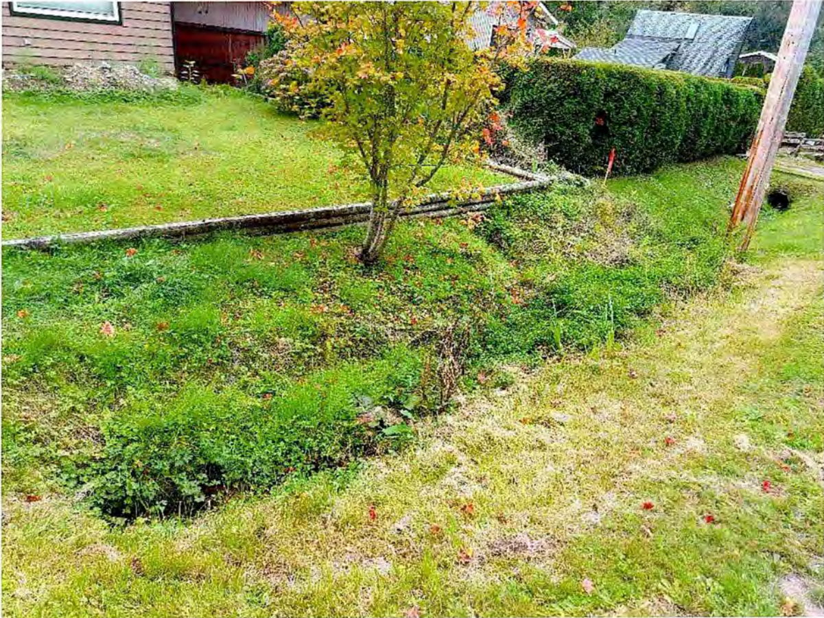
Photograph 2. Typical view of Ditch 1.
