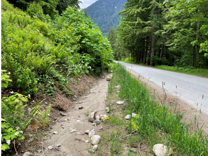
FIGURE 4-7: DITCH HAS BEEN INFILLED OVERTIME WITH SEDIMENT AND ROCK, REDUCING CAPACITY AND INFILTRATION CAPABILITIES
