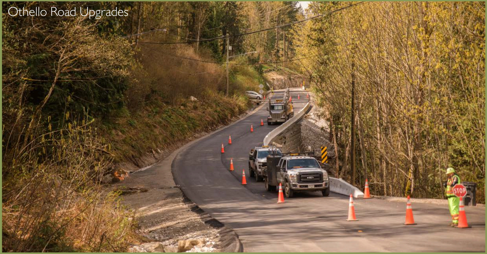
Othello Road Upgrades
