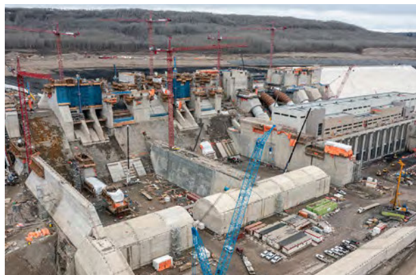
This aerial view shows Site C's spillways, penstocks, powerhouse and operations building for BC Hydro's third dam along the Peace River. Photo courtesy of Site C Team, BC Hydro.
