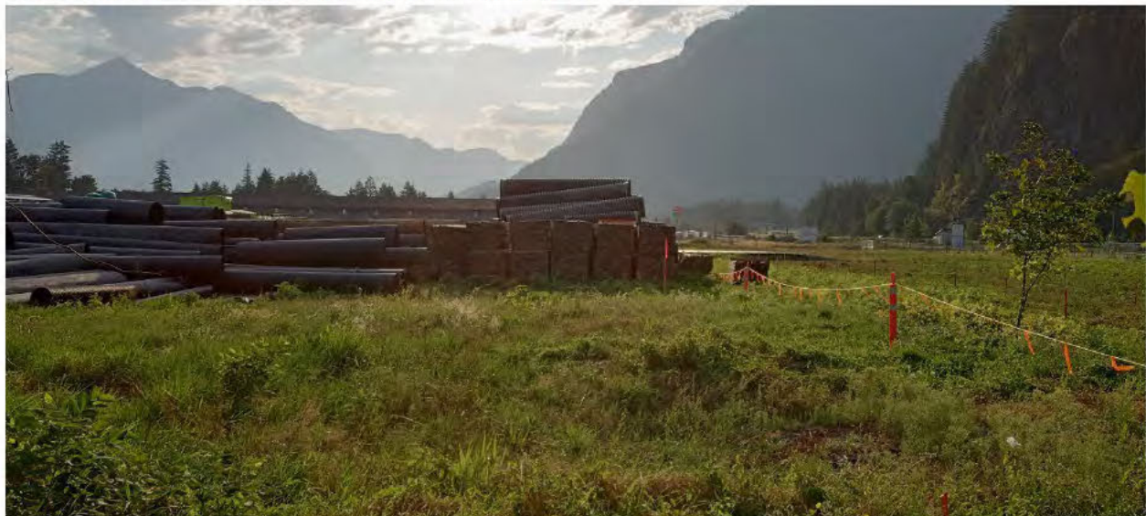
This is the pile of pipes that they dropped the other same sized pipe on to watch it bounce down to the ground shaking everyone's house really bad every time. Notice how high it is in comparison to the roof of the storage facility behind it. This is not as high as I have seen it.
