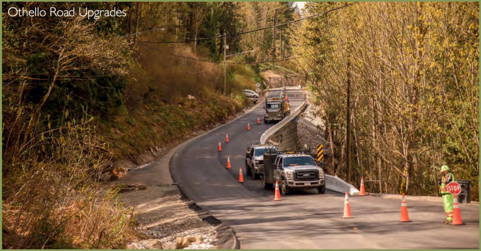
Othello Road Upgrades
