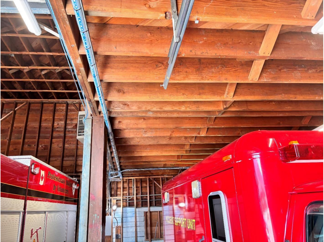
Figure 2 - Photo of underside of second floor. The 2 ply beam visible at the left side of the photo is beam F5 on the attached plans. The tall stud wall is visible at the left side of the photo in the background.
