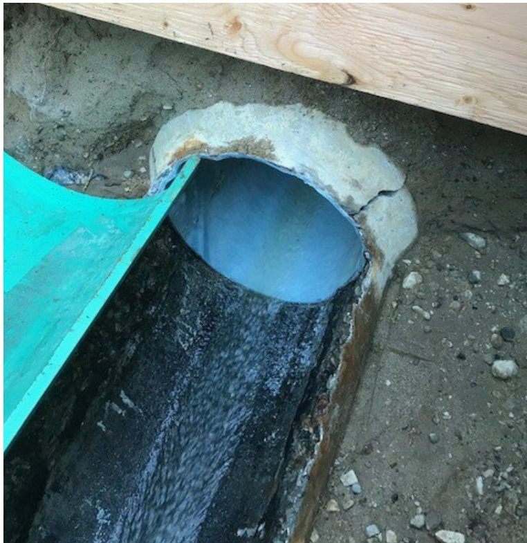
FIGURE 3-1: FRESHLY LINED FORCEMAIN
