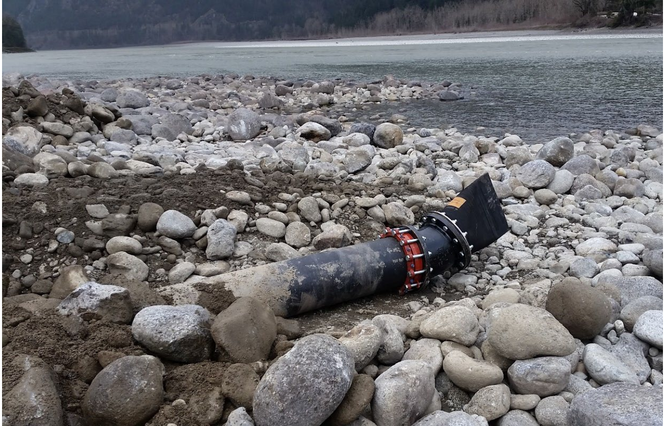
FIGURE 3-8: TEMPORARY OUTFALL AT TIME OF CONSTRUCTION
