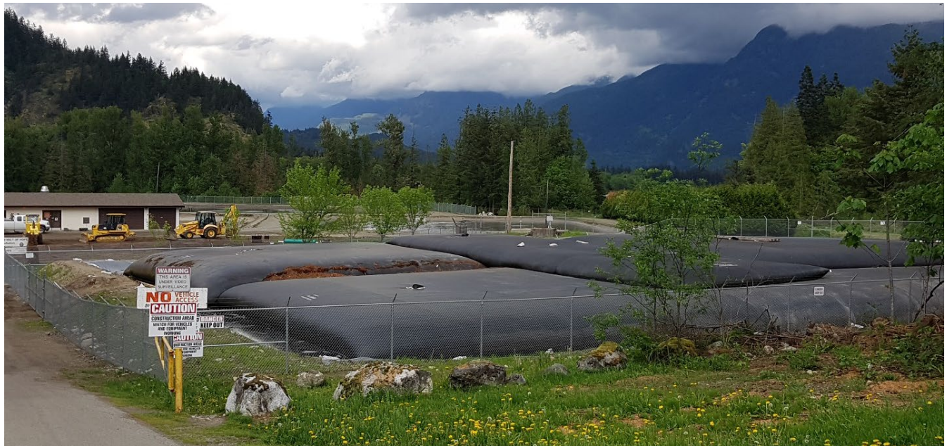
FIGURE 3-7: GEOTUBE BAGS CONTAINING SLUDGE REMOVED IN 2017.
