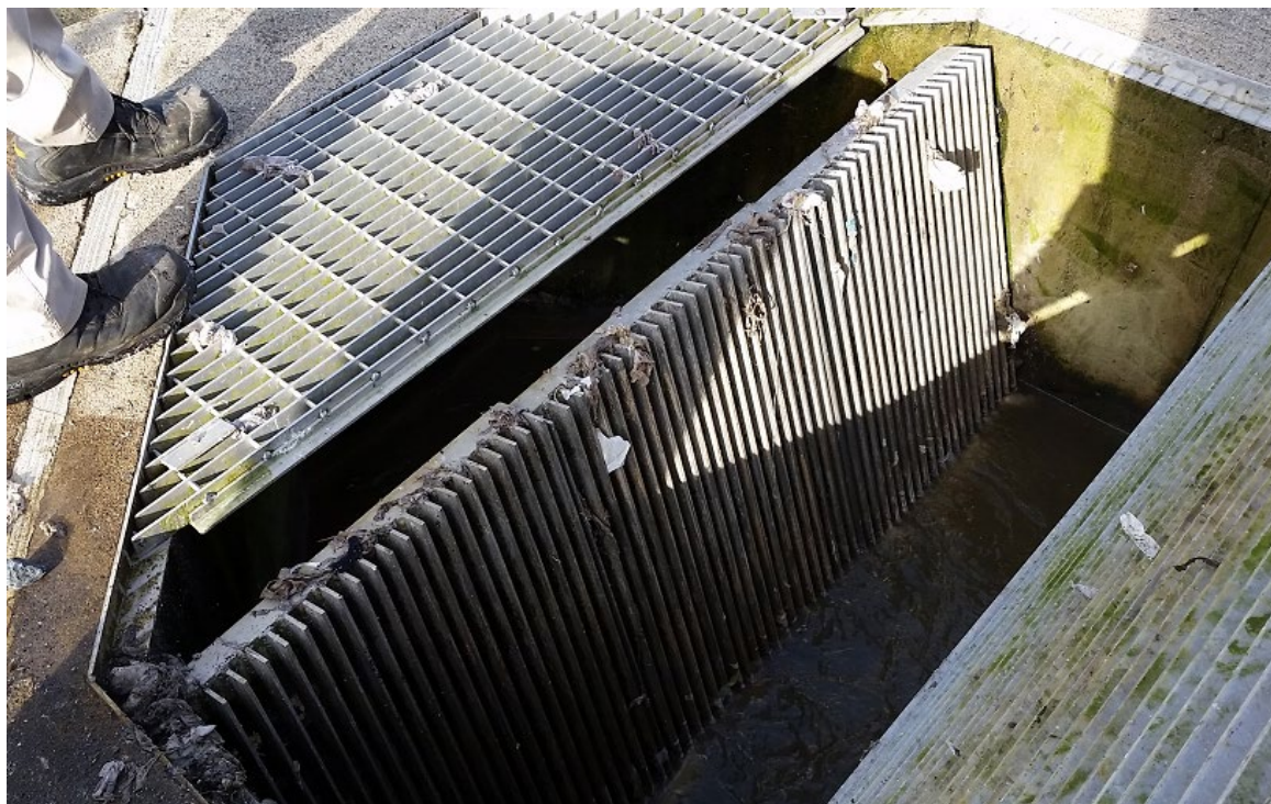
FIGURE 3-4: EXISTING BAR SCREEN
