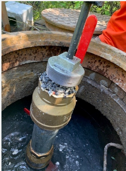
Removing a grease blockage from Tom Berry Lift Station
