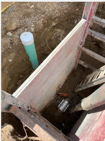
Sewer Main Repair
