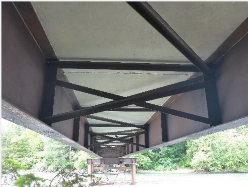
Golf Course Bridge Substructure
