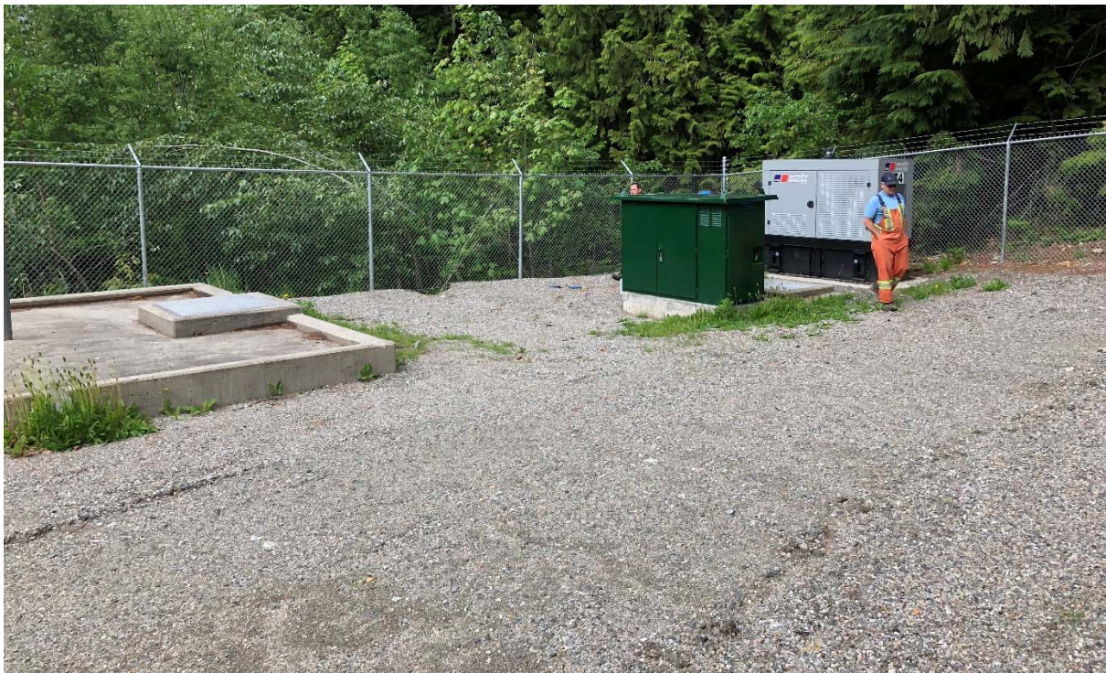
FIGURE 3-20: EAST KAWKAWA RESERVOIR
