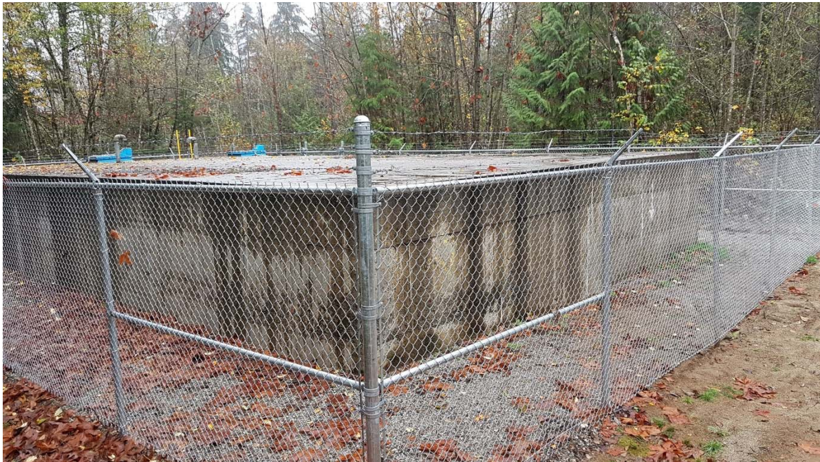
FIGURE 3-18: SILVER CREEK RESERVOIR
