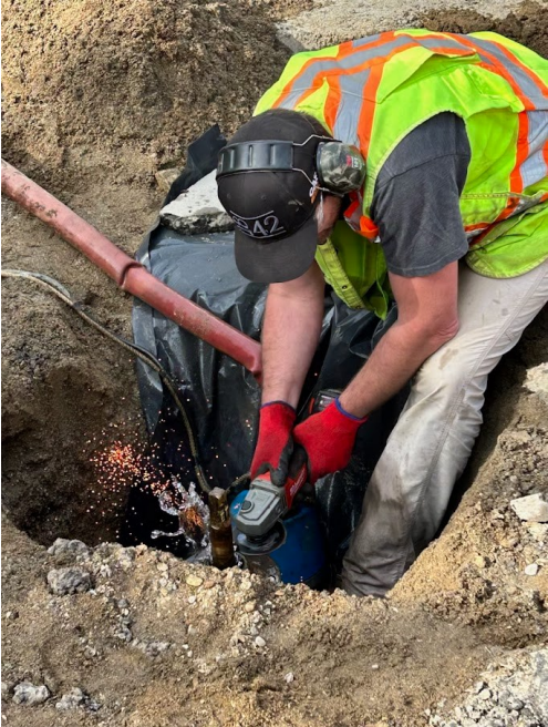
Leaking Water Valve Repair
