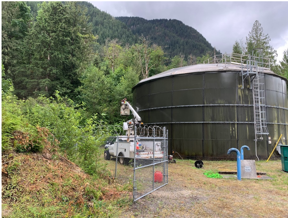
Cleaning of a Reservoir Tank
