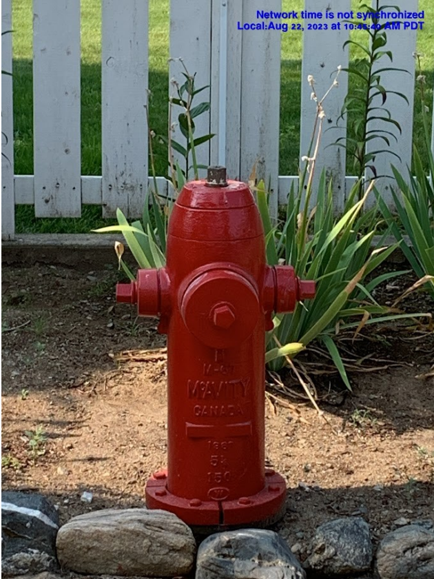
Freshly painted hydrant and pumphouse
